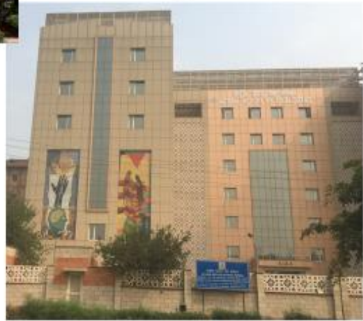
↓ Screened Roof top Utilities (After DUAC Observations compliance)
