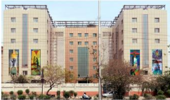
↑ Roof top Utilities visible (Before DUAC Observations)
